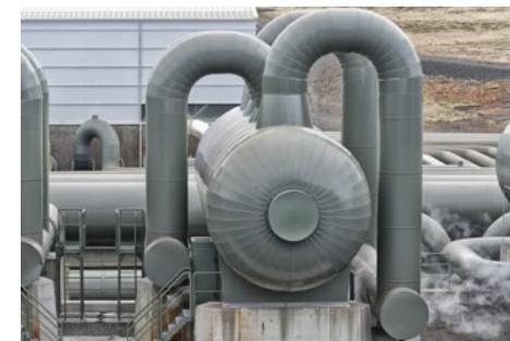
• the water supply pump station
